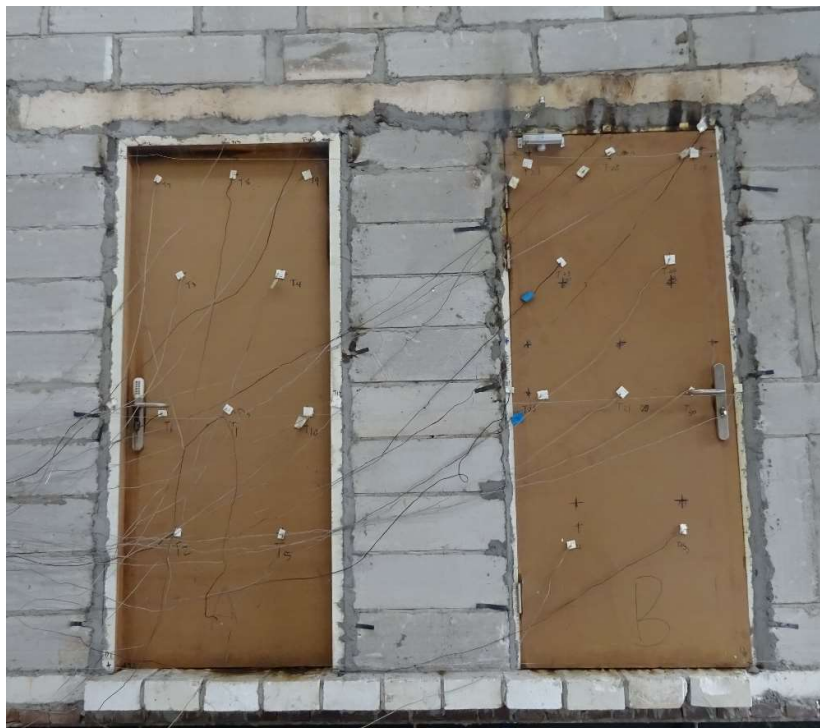
Photo No. 4 Unexposed Side after 40 Minutes
