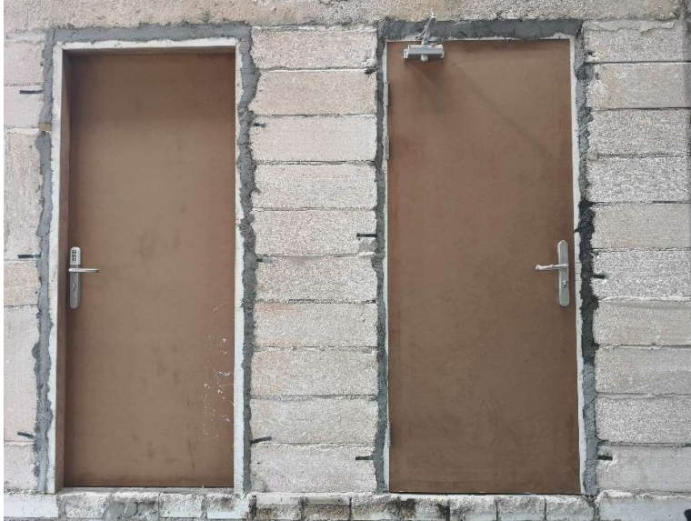
Photo No. 1 Exposed Side Prior to the Fire Test
